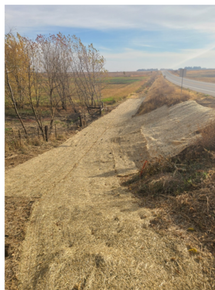
Erosion mats laid over disturbed soil
