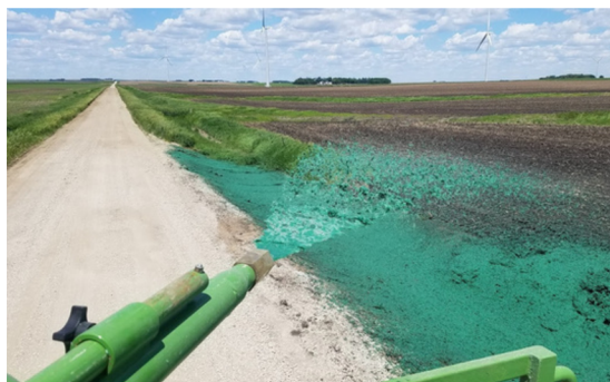
Applying hydromulch to a bare area of right-of-way
