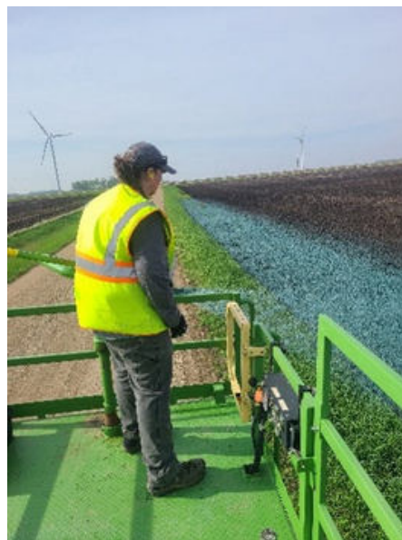
Hydroseed mixture (blue-ish green material pictured) sprayed into bare roadside
